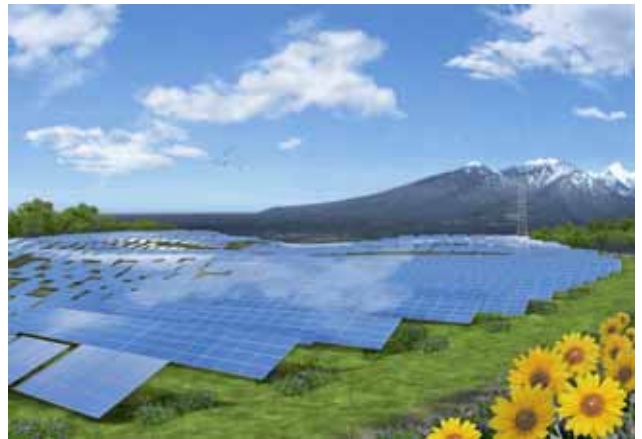
Fig. 12: Mega-watt photovoltaic system.
